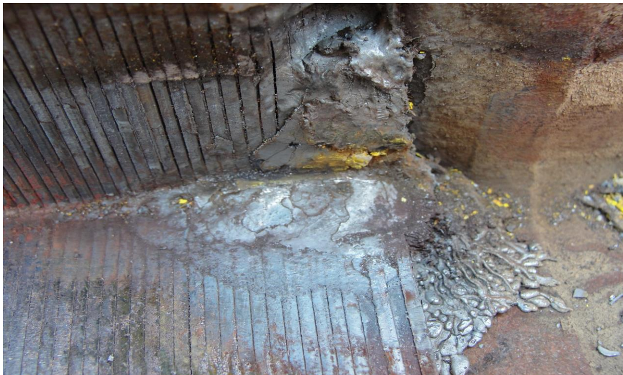
Figure 6. Melted field poles laminations
