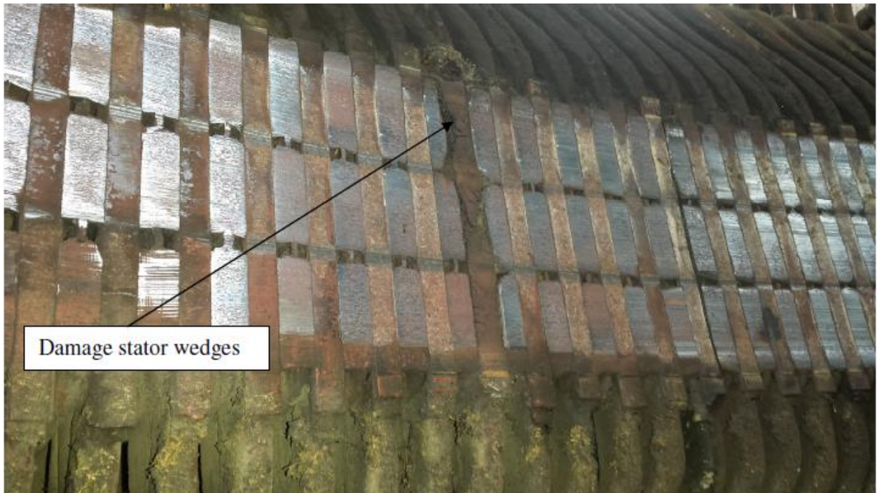
Figure 3. Damaged stator core iron and wedges
