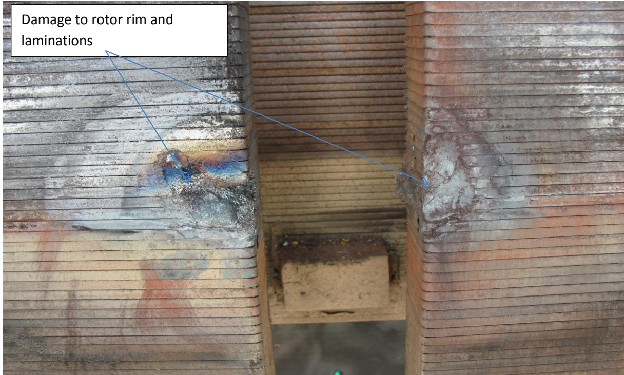
Figure 5. Damage to rotor rim and laminations
