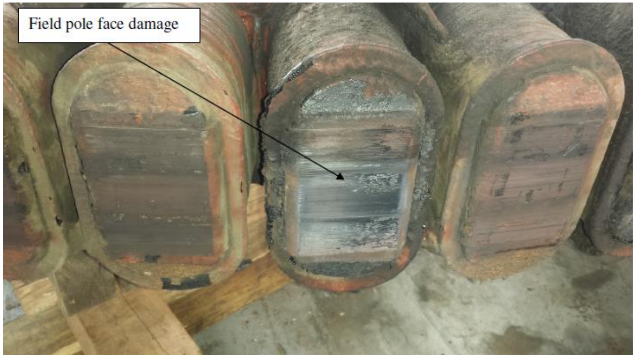
Figure 4. Mechanical damage to field pole face
